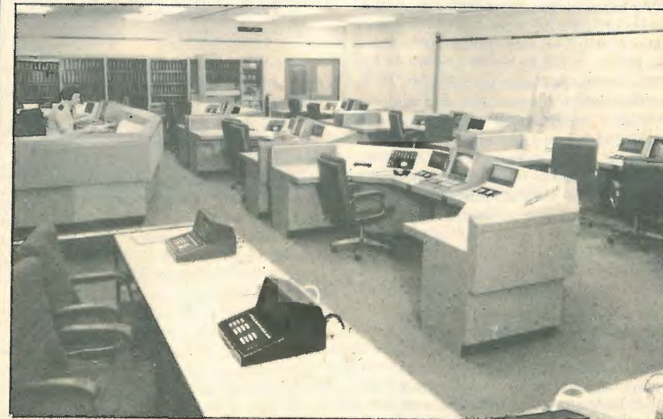
Main control room in the Leicestershire police communications centre.
